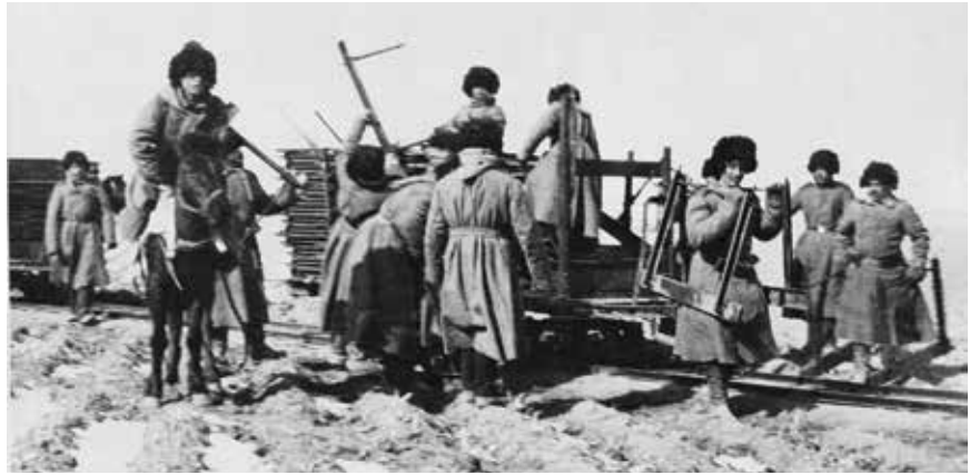
Russian army engineers seen here laying a track bed for a narrow gauge railway during the Russian campaign of March 1916 during World War I. (DAILY MIRROR ARCHIVE/MIRRORPIX/GETTY IMAGES)
