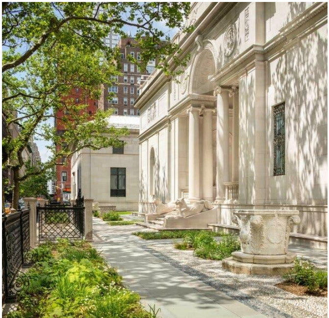
Recently renovated Morgan Library exterior.
